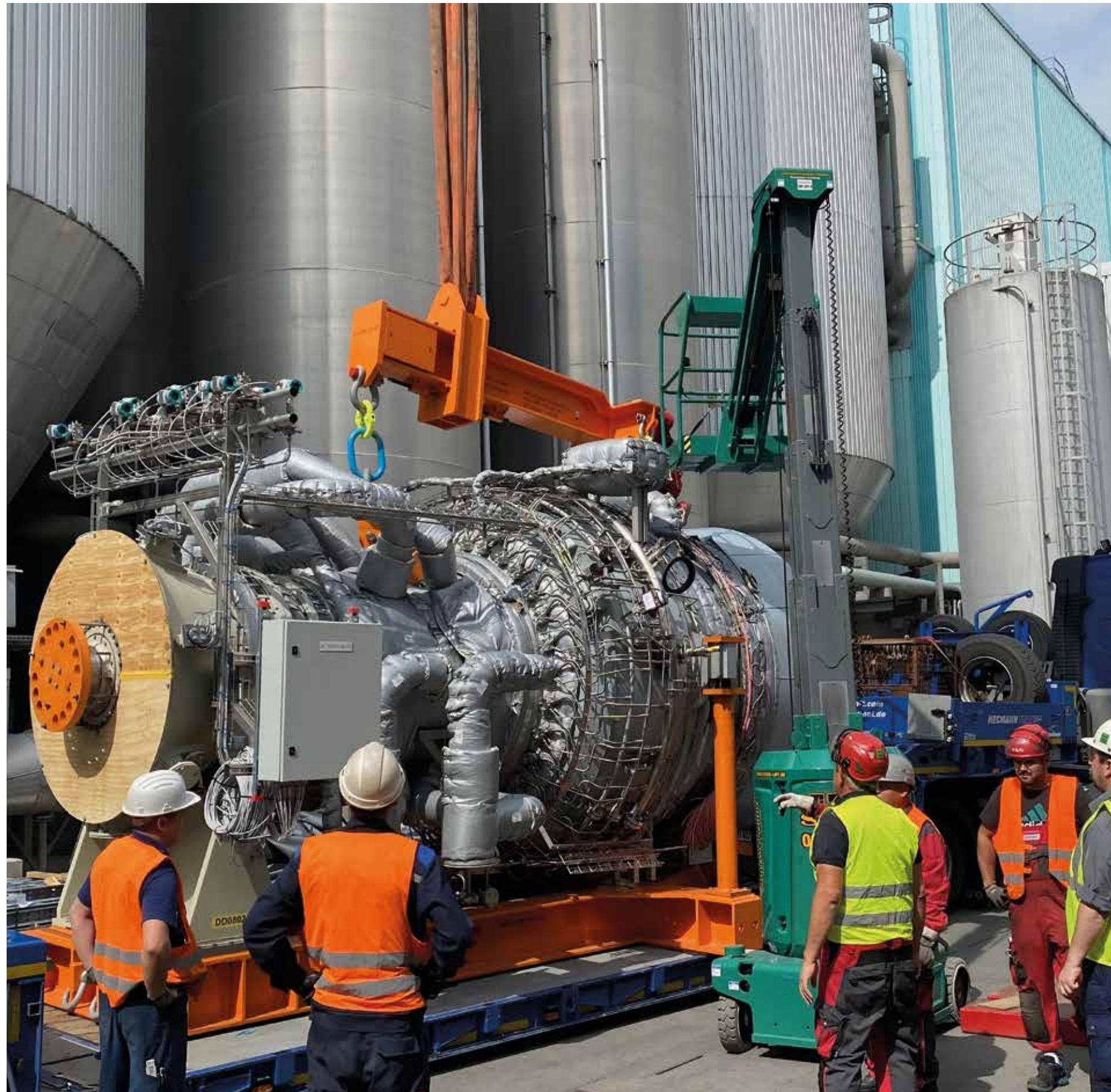
Delivery of the new gas turbine at Papierfabrik Palm in Eltmann. PALM is the first company in the world to use the latest generation of gas turbines in three of its power plants – already today they are able to run on up to 75 % green hydrogen.
