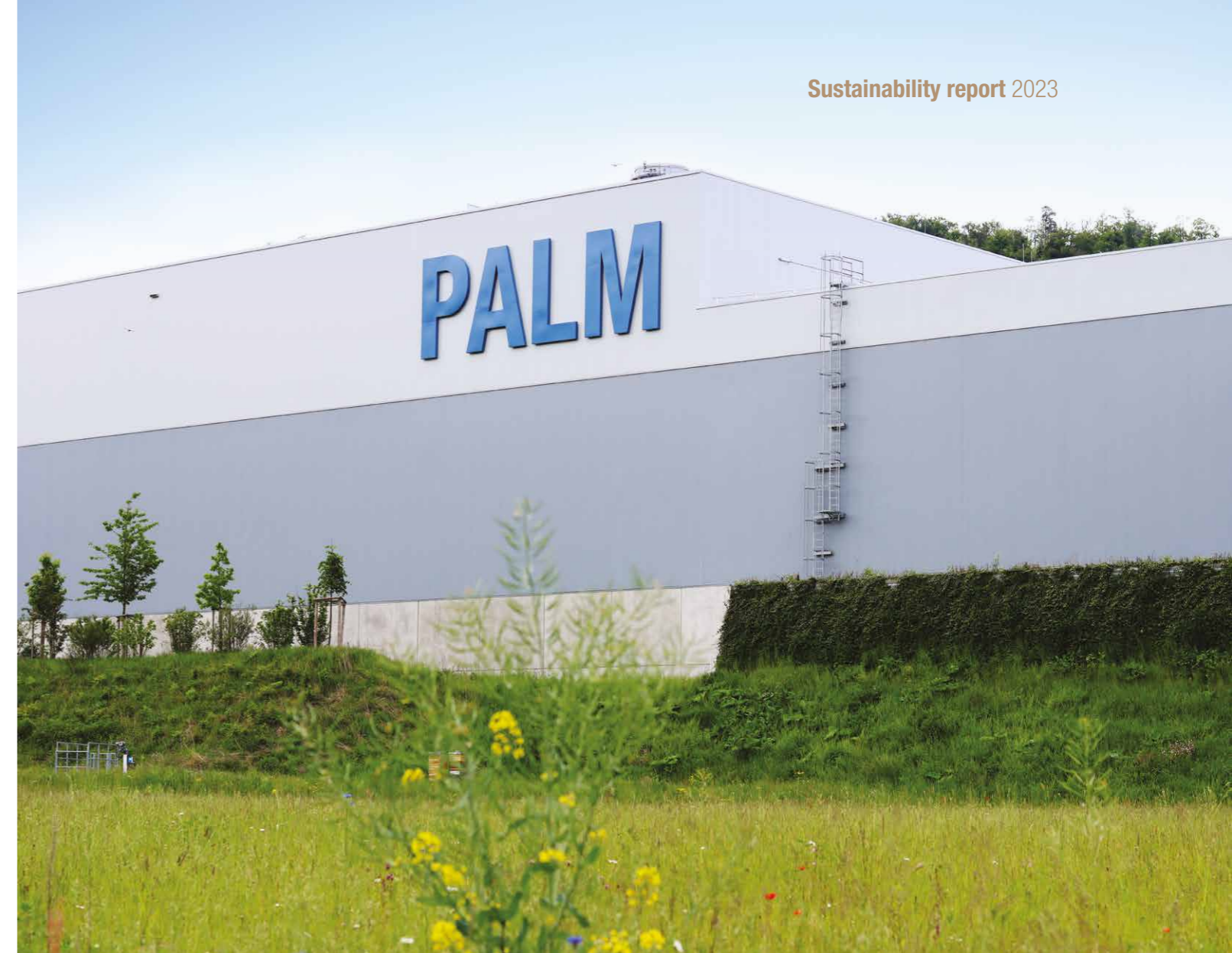
Renaturalised area and newly created wildflower meadow on the mill premises in Aalen.
